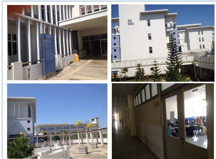
Figure 1-2 The Faculty Engineering's Common Classroom Building
