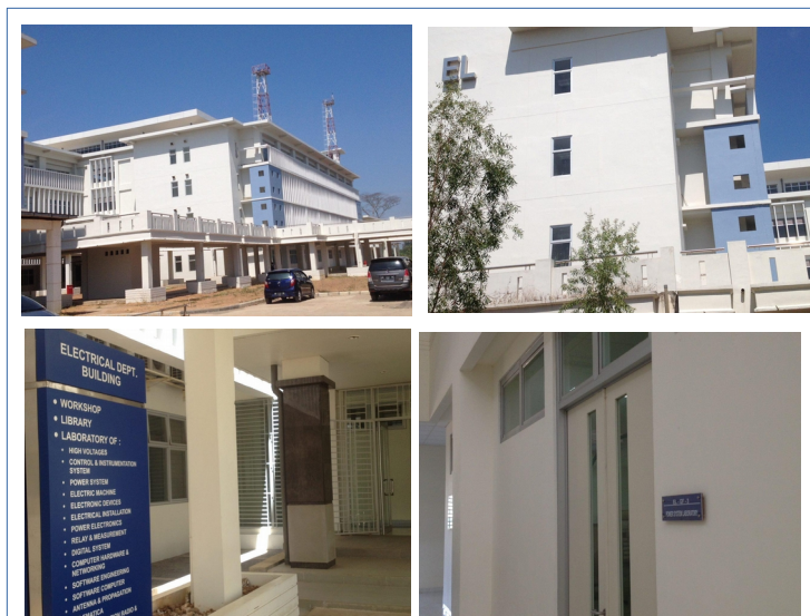
Figure 1-3 The Electrical Engineering Building
