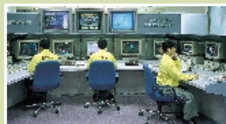
The total building management service BOSS-24 uses remote monitoring and control via communications circuits to permit semi- and fully-automated building management.
