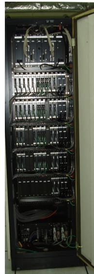
Gambar 6.04. *EFCD Duplexed Field Control Station*
