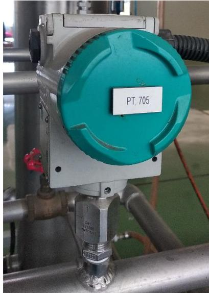
**Gambar 2.20 Pressure Transmitter**
