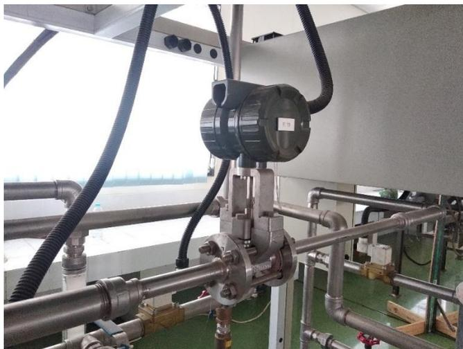
**Gambar 2.8 Vortex Flowmeter Transmitter**
