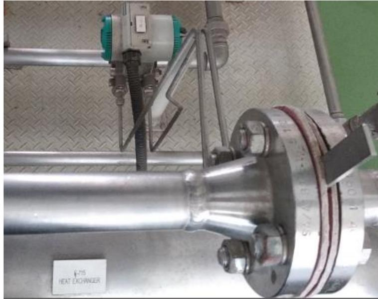
**Gambar 2.10 Orifice D/P Transmitter**
