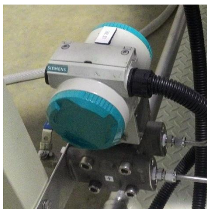
Gambar 2.15 Water Level Sensor
