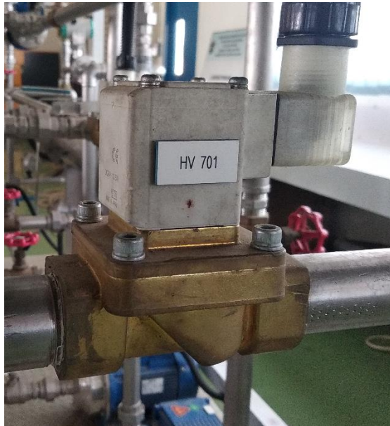
Gambar 2.16 Selenoid Valve
