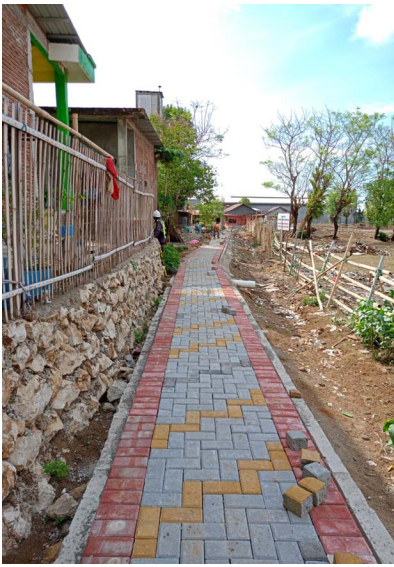
Paved pathways and drainage
